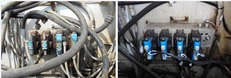
*Four hydraulic valve replacement on manifold, re-routed plumbing and rewired - before (L) and after (R)*
