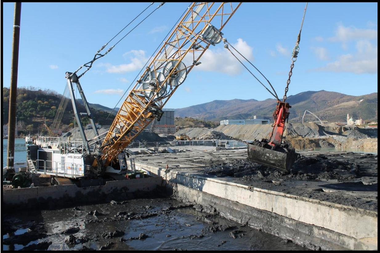
*In the Port of Vado Ligure the HS 8130 HD removes the sediments with a hydraulic clamshell bucket.*
